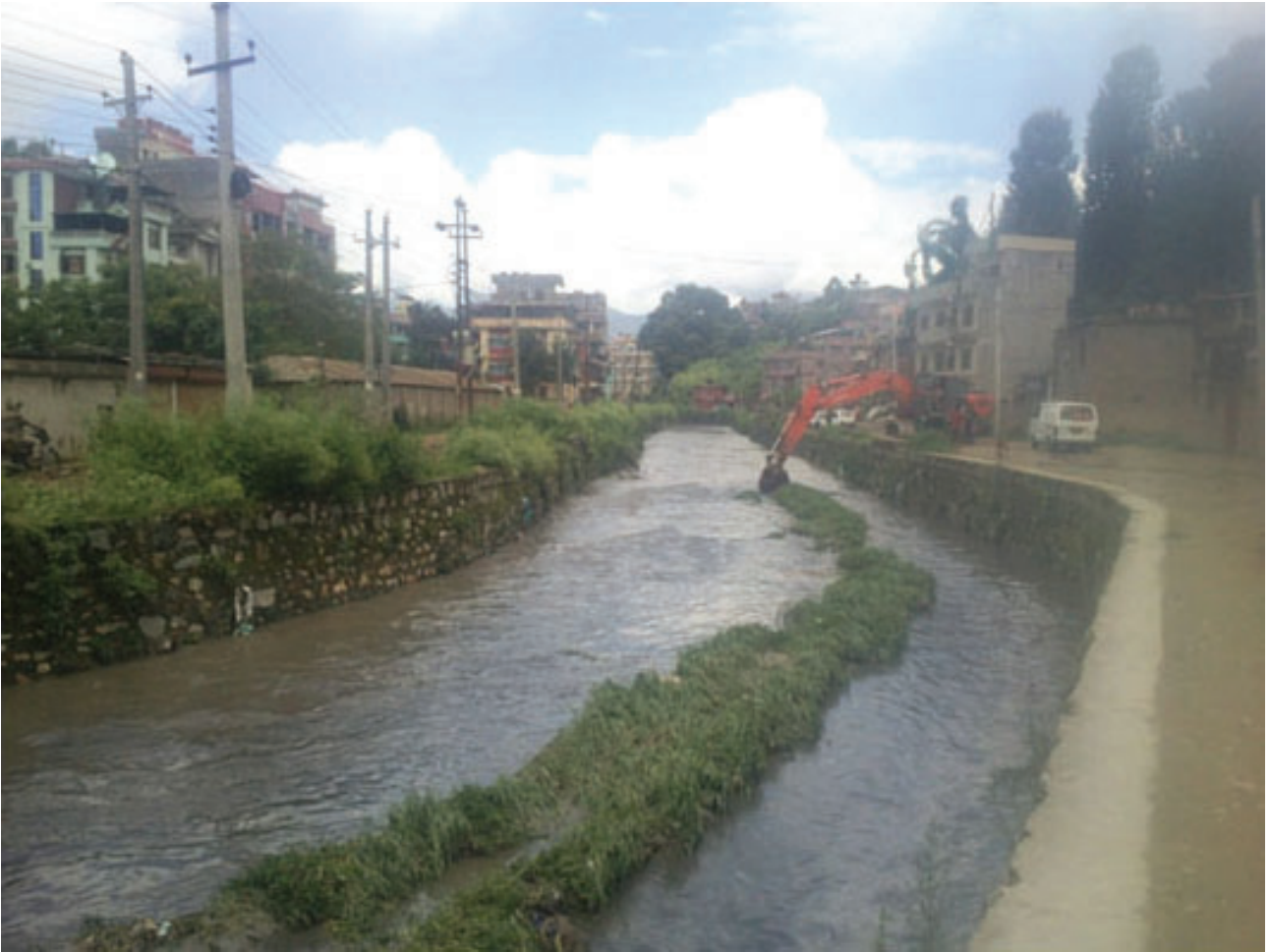
Figure 26: River cleaning at Baneshwor
