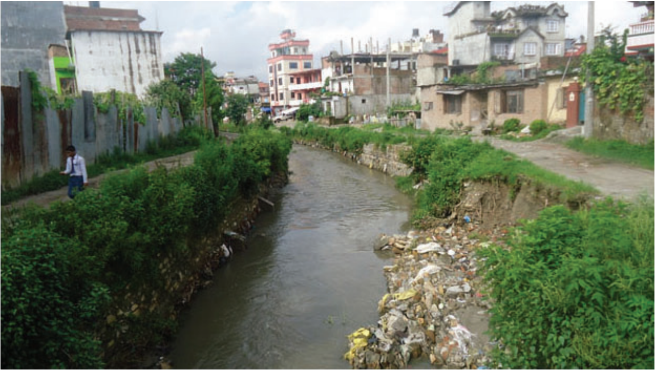
Figure 17: Damage done by Dhobikhola due to flooding
