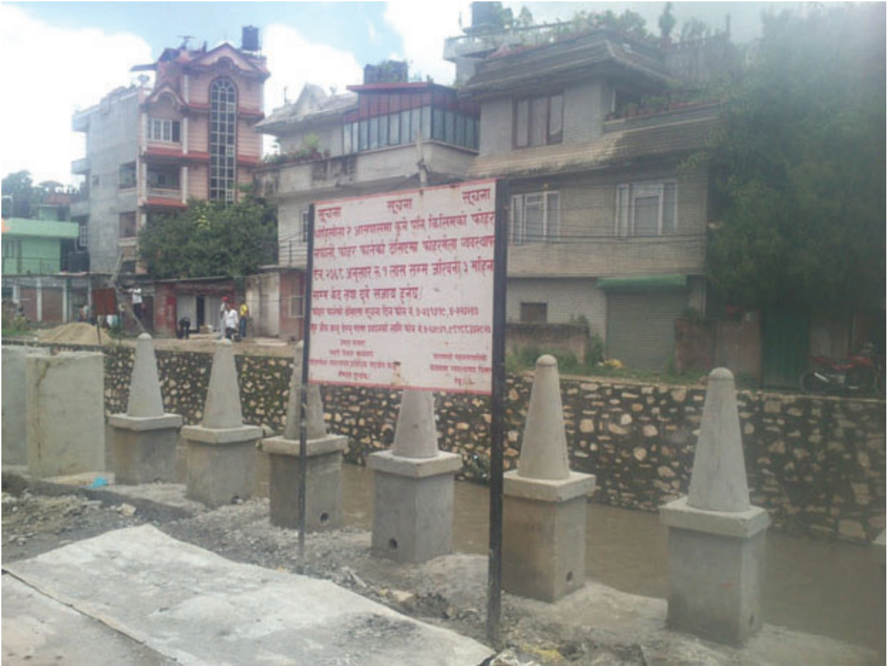
Figure 24: Awareness board and road under construction at the bank of Dhobikhola
