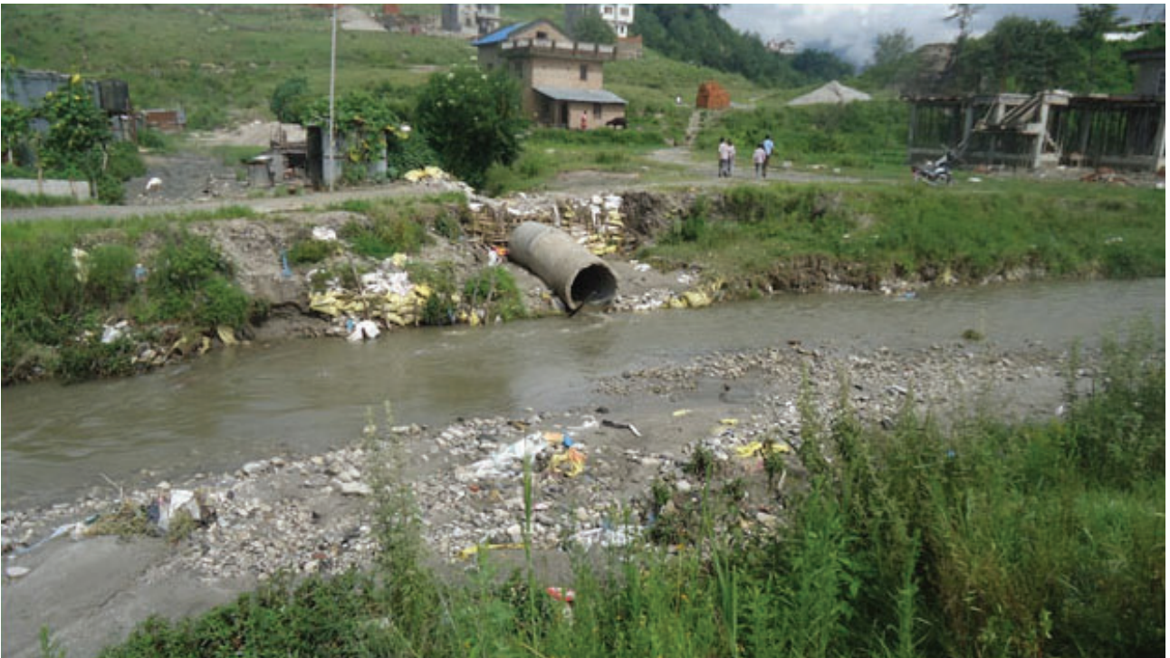
Figure 11: Opening of sewer pipe at Dhobikhola
