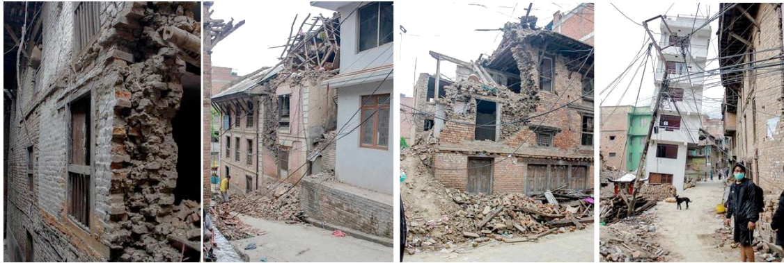
Figure 3: Damage Level due to Earthquake in Panga
