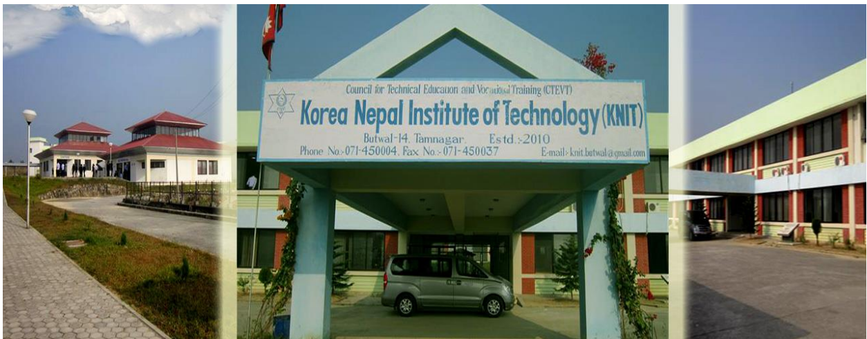
Figure 3 KNIT building, Tamnagar, Butwal
