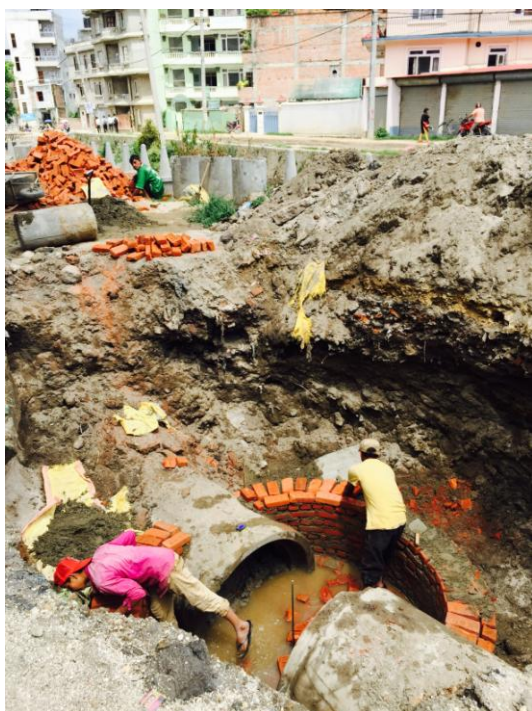
Figure 3: Sewer pipe being constructed near Bijulibazar area.
