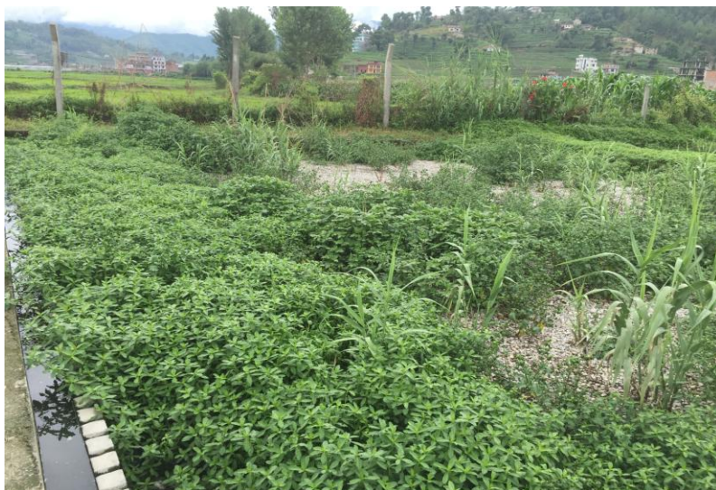
Figure 6: Sreekhandapur wastewater treatment plant in Sreekhandapur, Dhulikhel.
